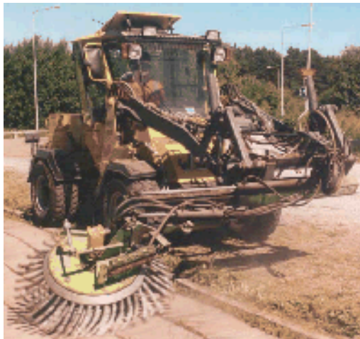
© City of Göteborg (Mechanically operated brushing machine)
